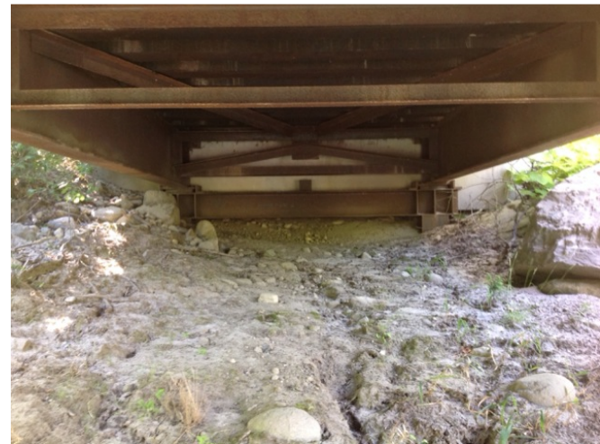
Right Bank Abutment when facing downstream
