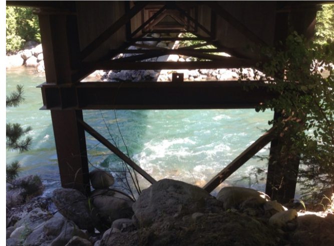
looking at pier from woods end
