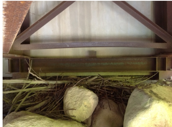
left abutment bearing
