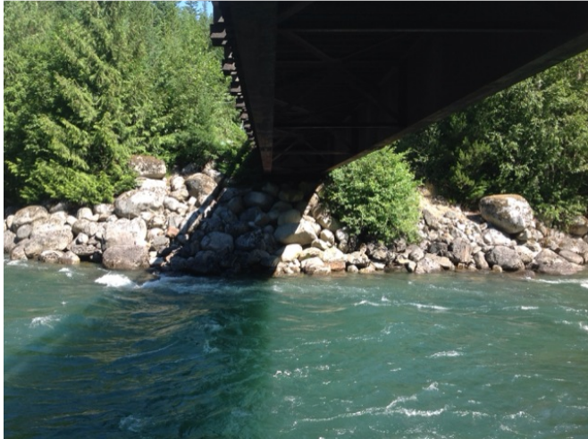
Left Bank Abutment when facing downstream
